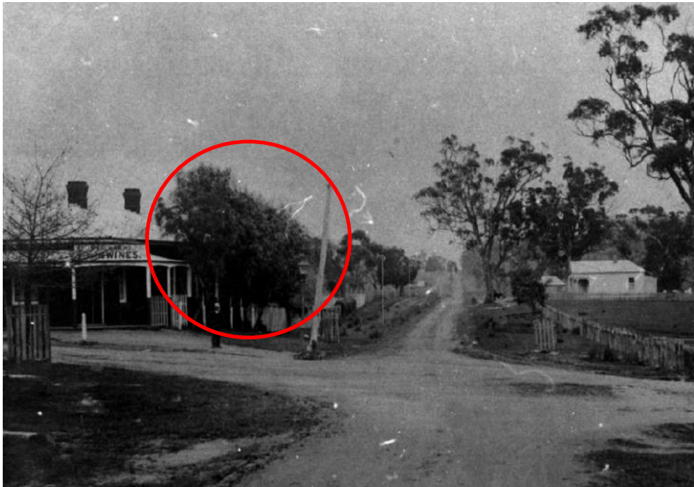
Figure 5 Deschamps Wine Store and Olive trees at 2-4 Albert Hill Road, Lilydale
